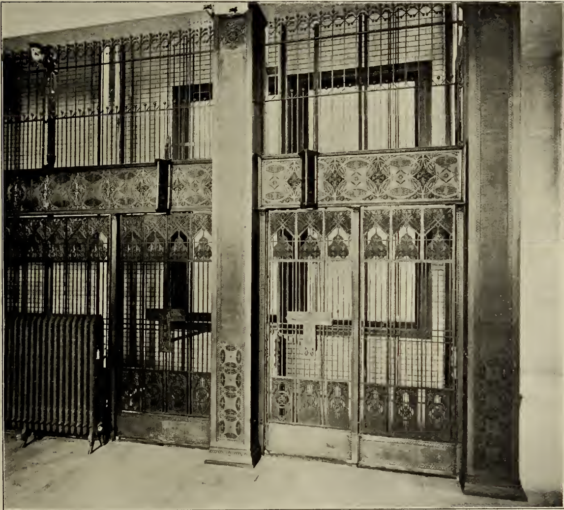
ELEVATOR INCLOSURES, UPPER FLOORS, CHICAGO STOCK EXCHANGE.
